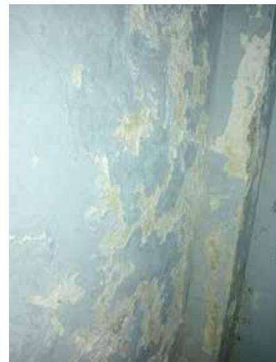
Fig 4 & 5 Show occurrence of salt action
