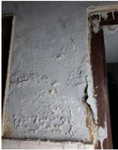
Fig 3 & 4 Show the penetration seepage
